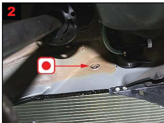
2 Wheel arch rear/rear wing: Treat via existing plugged hole.
