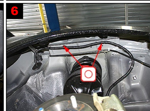
6 Wheel arch front top member: Treat via existing holes.
