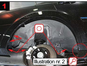
1 Wheel arch rear/longitudinal member: Treatment via 1 drill hole and existing holes. Panel: Fig 2.
