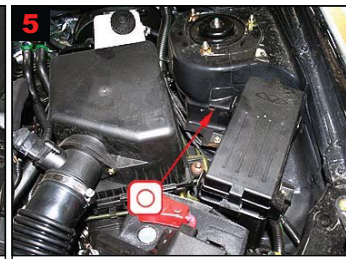
5 Engine compartment - sectional view: Reinforcement on spring strut left side. Treat via existing hole.
