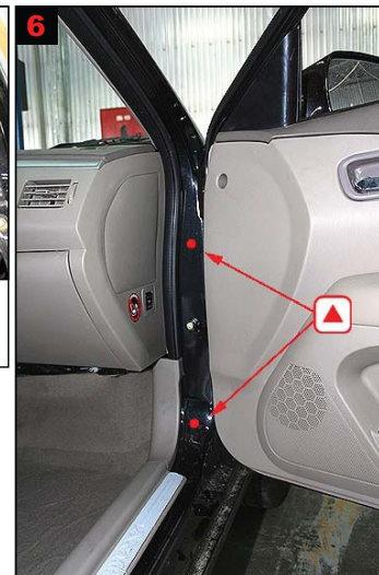
6 A-pillar: Treat via 2 drilled holes.
