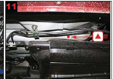
11 Longitudinal members centre above tank: Treat via 1 drilled hole each side.
