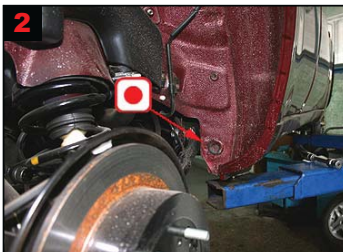
2 Wheel arch rear/panel: Treat via existing plugged hole.
