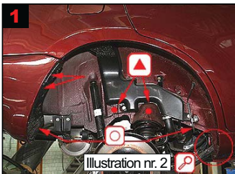
1 Wheel arch rear/longitudinal member: Treatment via 1 drill hole and existing holes. Reinforcement for spring: Treat via 1 drilled hole. Panel: See fig 2.
