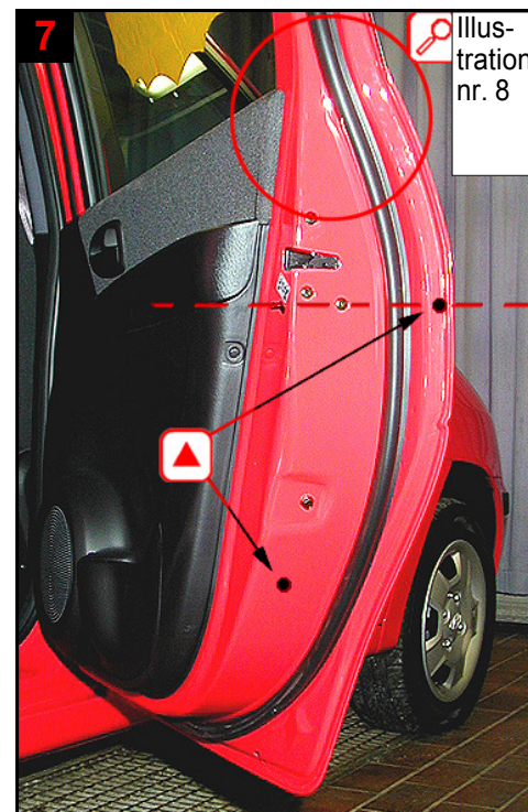
7 Illustration nr. 8 Rear door: 3 drill holes for correct treatment. See fig 8 for drilling behind rubber strip.
