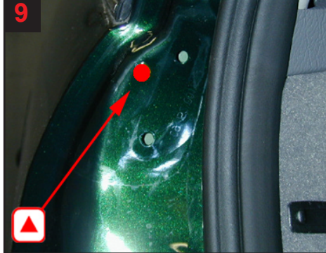
9 C-pillar. Remove rubber strip, Treat via 1 drilled hole.
