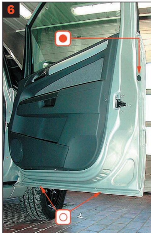
6 Front door: No hole according to dealer because of airbag. Treatment via existing plugged hole and drain holes in bottom.
