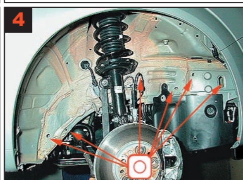
4 Wheel arch front/longitudinal member: Treat via existing holes and gaps.
