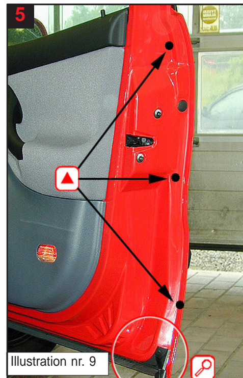
Front door: Treat via 3 drilled holes.
