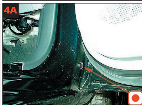
4A A-pillar: Treat via existing plugged hole.
