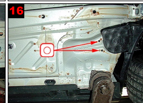
16 Small cross member after front wheel arch: Treat via existing holes.
