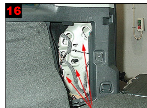
16 Rear wing from boot: Treatment via existing lug by tail light, treat with caution in all directions.
