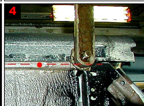
4 Panel sectional view: Fig: drilling at correct level.
